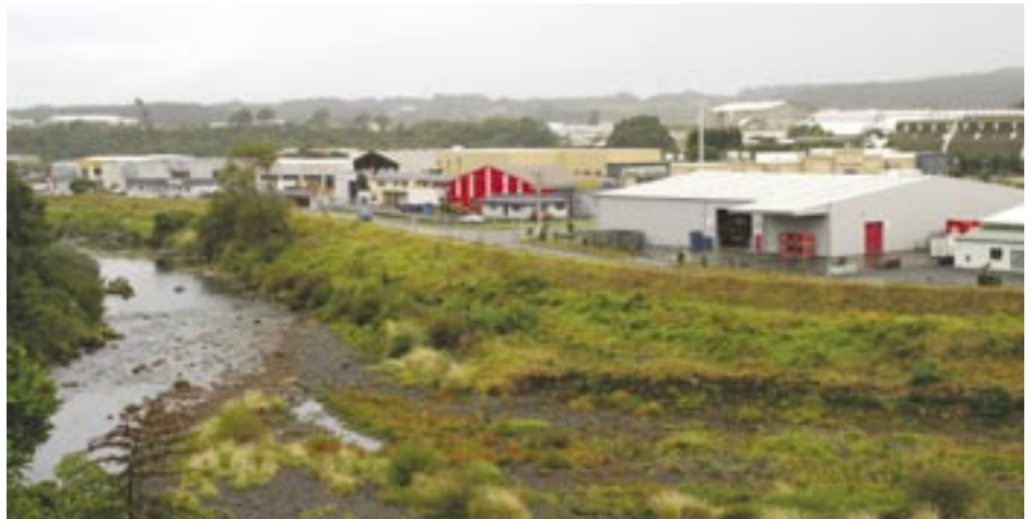
Management of the Lower Waiwhakaiho area has ensured good environmental performance.
