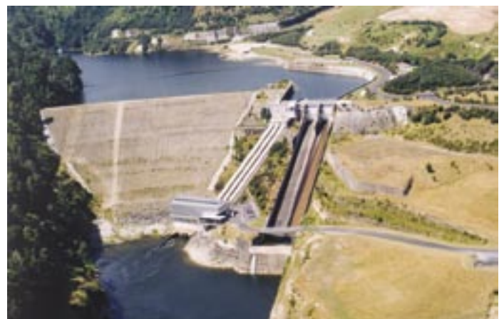
Patea hydroelectric power scheme
