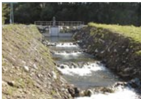
The new fish pass at the Motukawa Power Station is designed to accommodate the new residual flow from the hydroelectric scheme.
