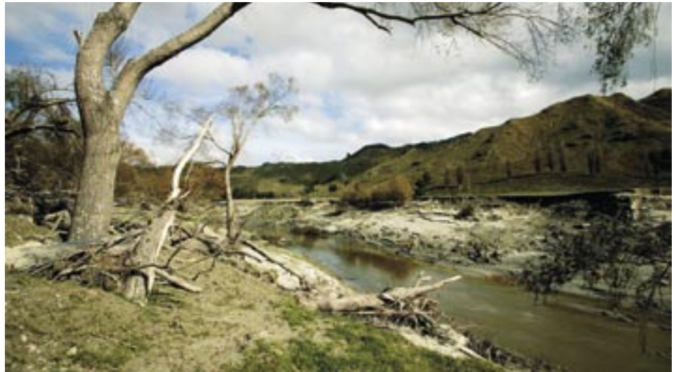
Slumping of Waitotara river banks seen two months after the flood.
