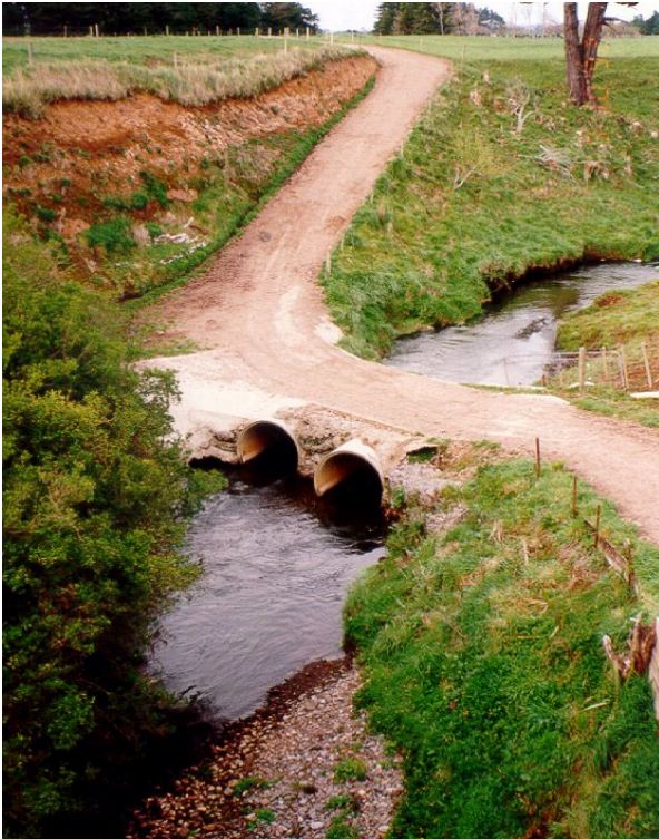
Figure 7: Stream bridge or culvert
