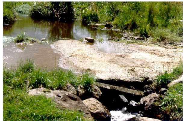
Figure 6: Concrete or gravel stream crossing
