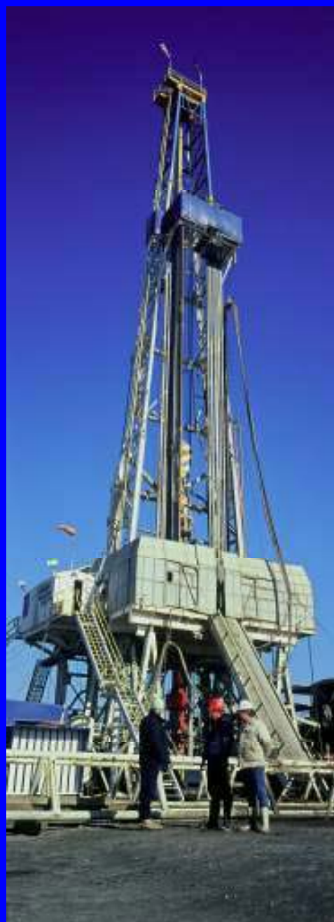
Photo 1: A petroleum exploration drilling rig in Taranaki
