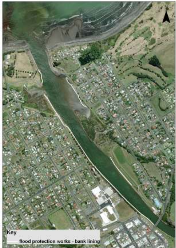
Figure 1: Waitara Flood Protection Scheme – downstream of the Town Bridge
