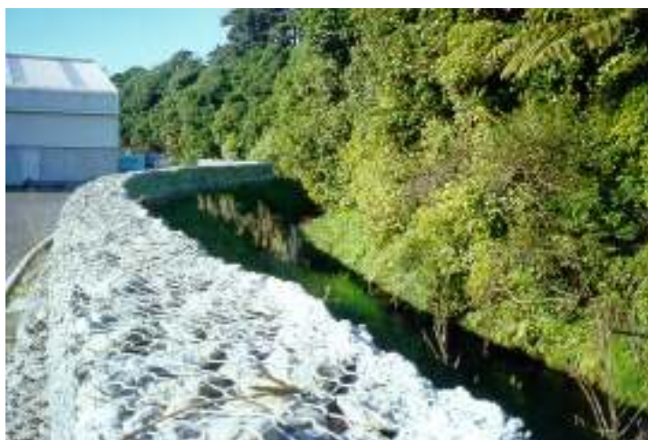
Mangaone flood defence wall
