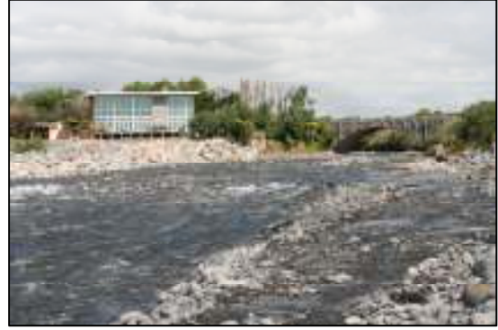
Stony River – completion of works
