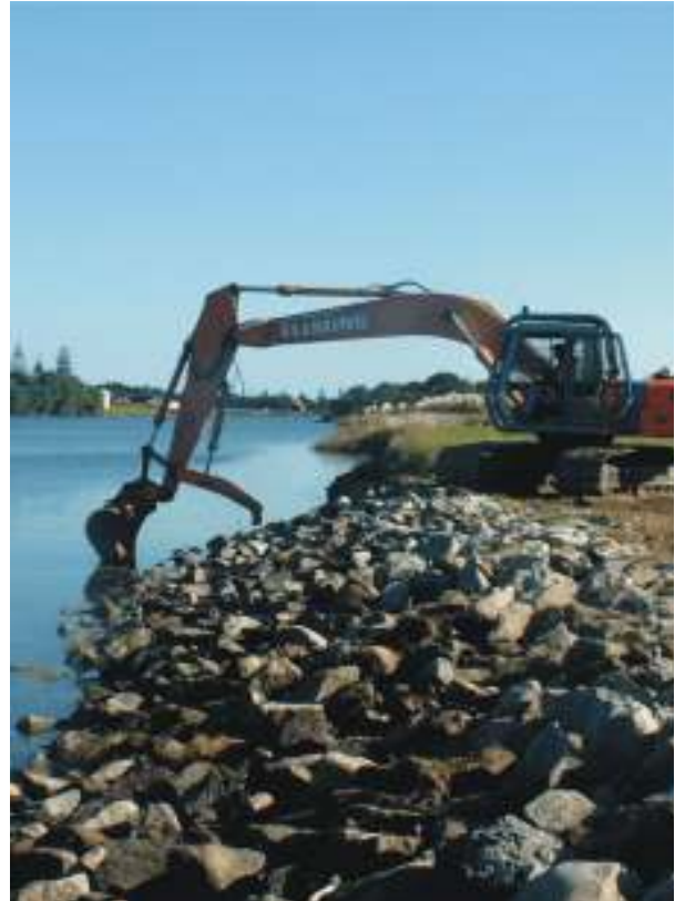
Bank protection rock works associated with the Waitara Flood Protection Scheme
