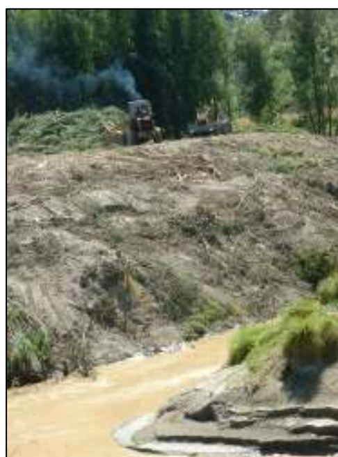
Channel clearance – Waitotara River
