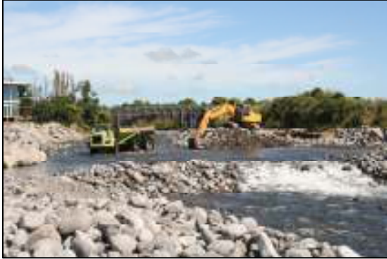
Stony River – work in progress
