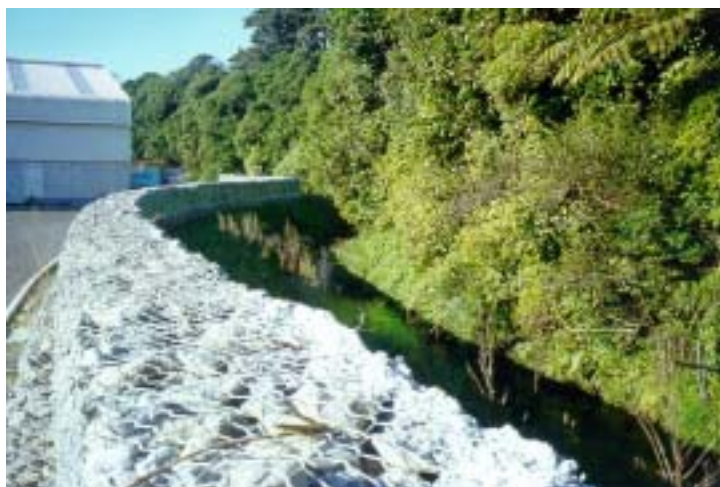
Mangaone flood defence wall
