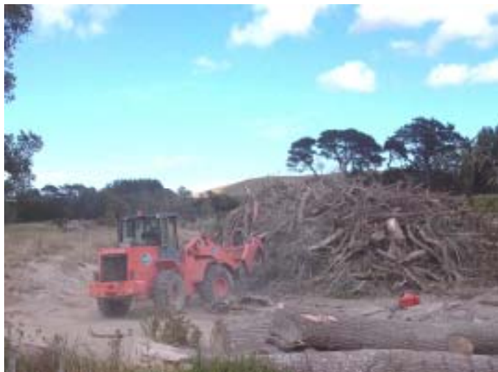
Mechanical channel clearance of vegetation debris in the Waitotara catchment
