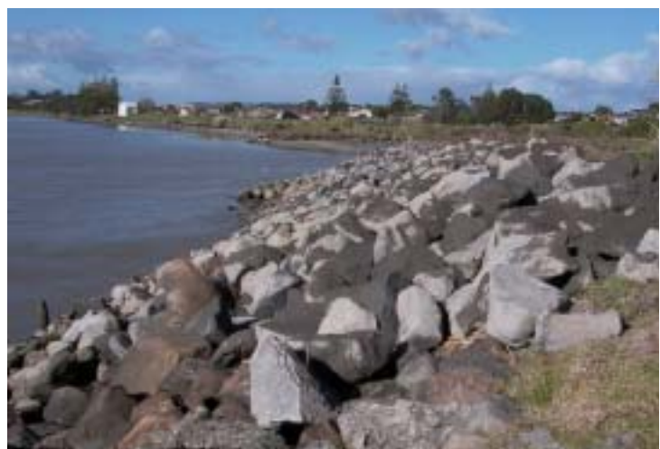
Rock bank lining
