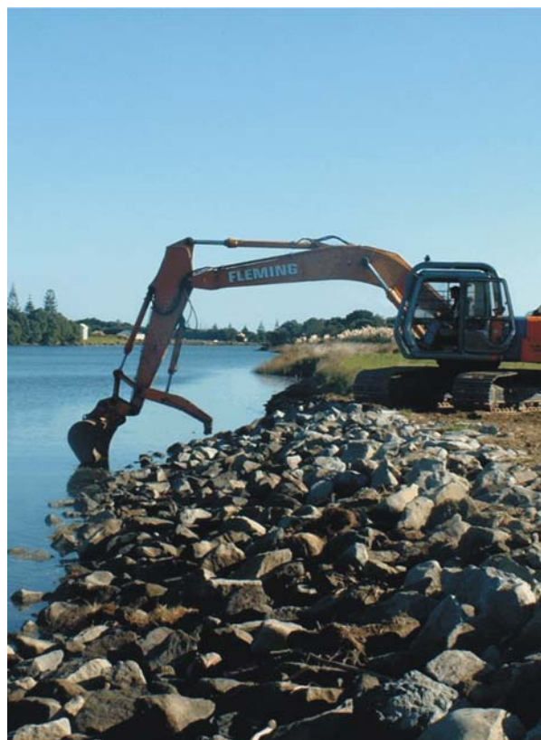
Bank protection rock works associated with the Waitara Flood Control Scheme
