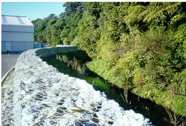
Mangaone flood defence wall
