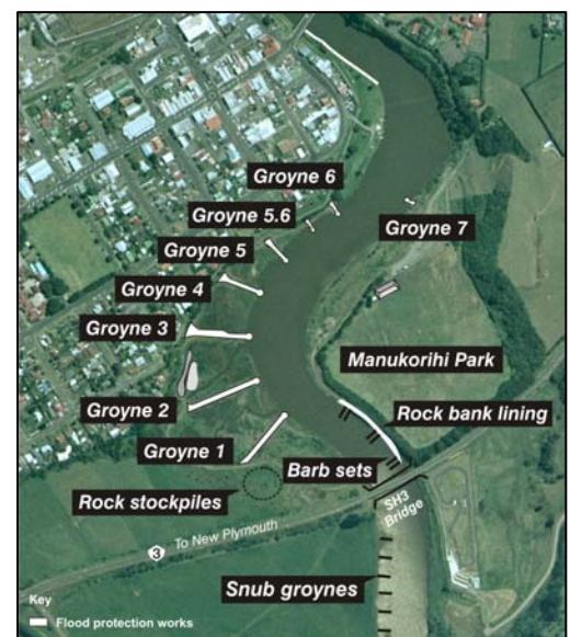
Figure 2: Waitara Flood Protection Scheme - adjacent to the Town Bridge
