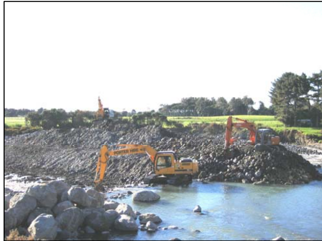
Stony River downstream of SH45 Bridge
