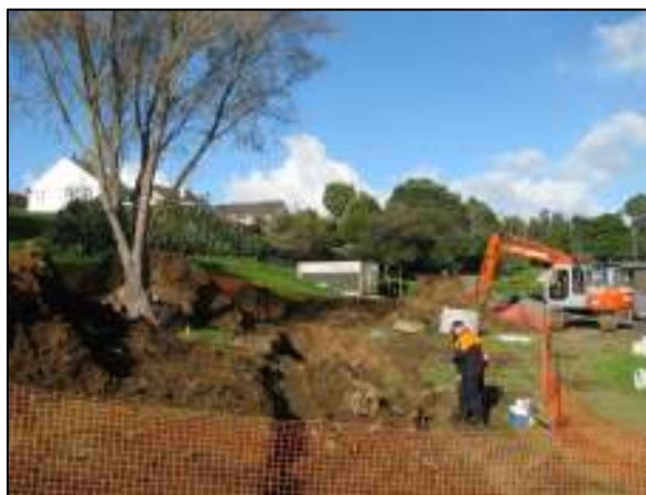
Laying of stormwater pipes excavated crushed drums
