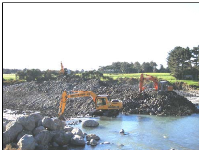
Stony River realignment downstream of SH45 bridge
