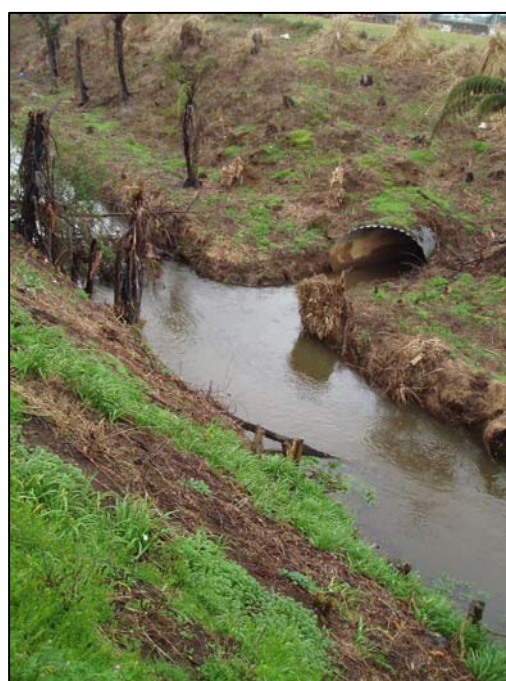
Channel clearance Mangaone Stream
