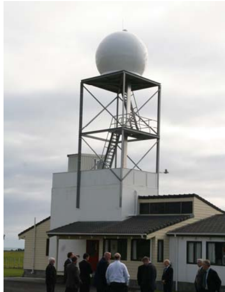
Photo 6: Councillors & senior staff inspect Met Service weather radar at New Plymouth Airport
