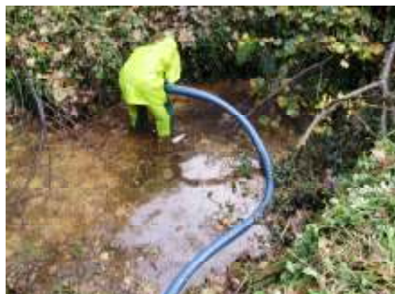
The cleanup of the discharge from Caltex, Stratford
