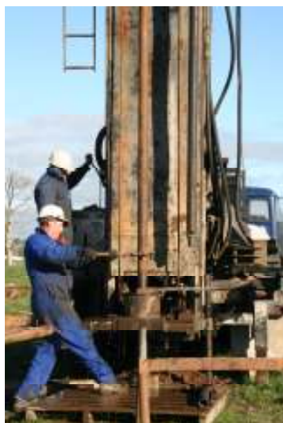
Water bore drilling in South Taranaki
