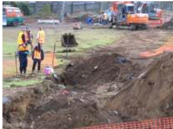
The Marfell Park cleanup operation
