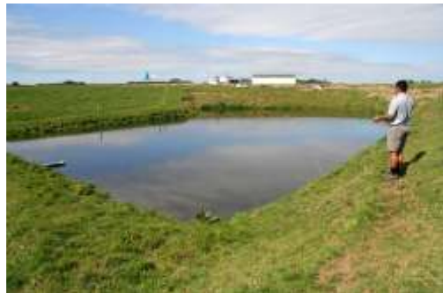
Oxidation pond annual inspection
