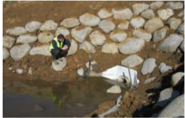
A Council officer checking the installation of a culvert
