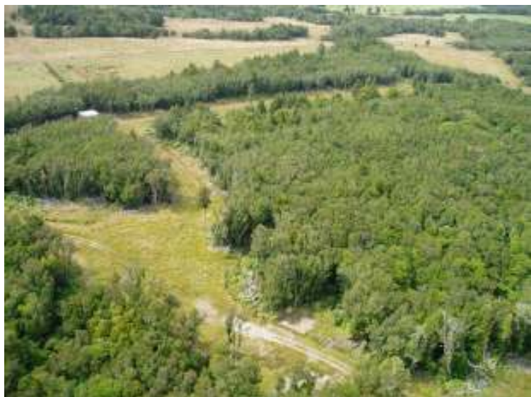
Vegetation clearance and land drainage activities at the Alfred Road Wetland
