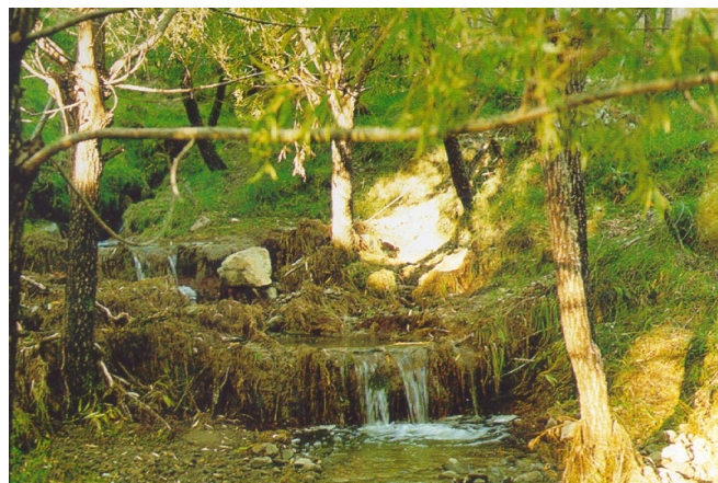
Fig. 2 Stabilisation planting next to debris dam
