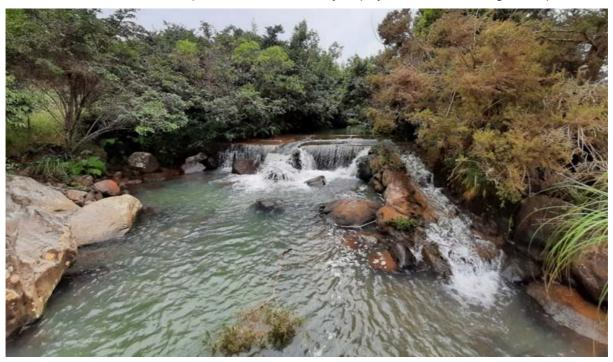
Photo 1 STDC weir, new fish pass (right of photo) and old degraded fish pass (centre of photo) in the Mangawhero Stream 2022. A small perch out the downstream end of the ramp is present
