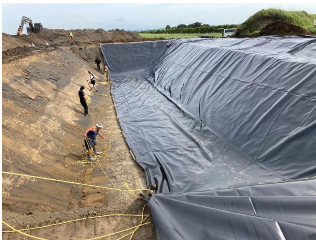
Pit 2 Liner installation.
