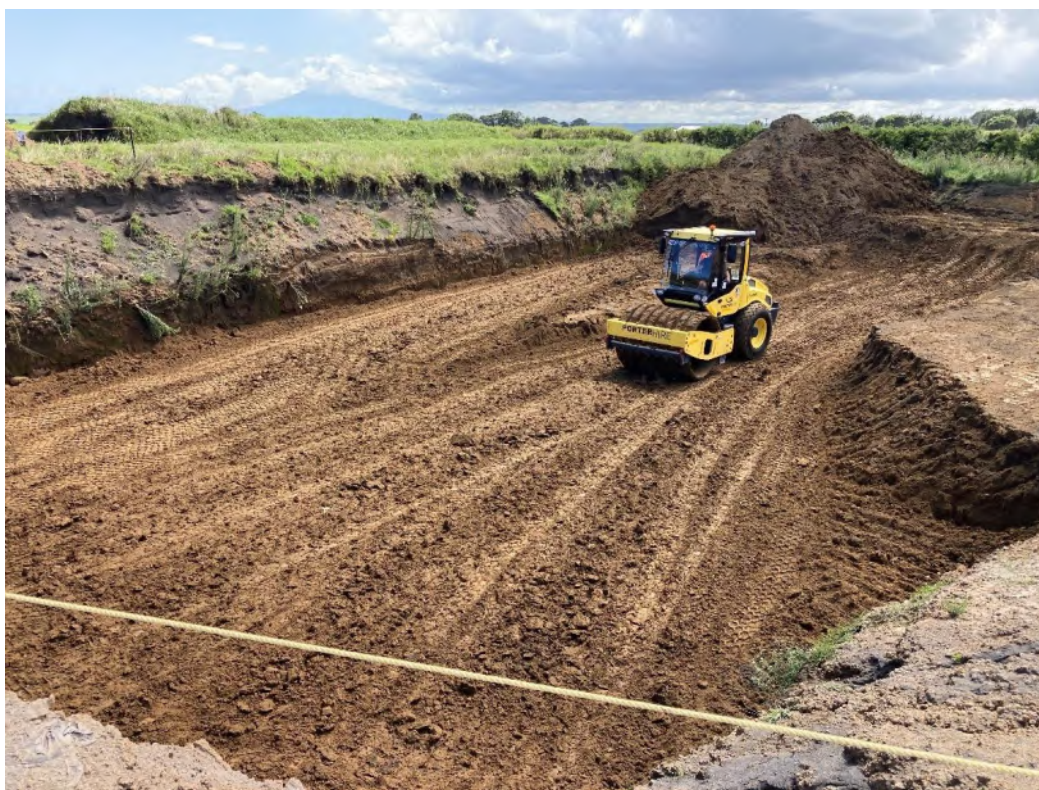
Pit floor Construction/Compaction.
