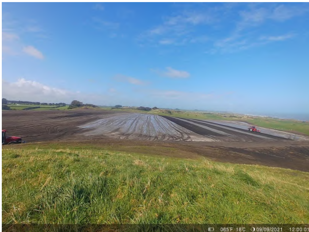
Spreading/Deep Ripping Incorporation into Sands
