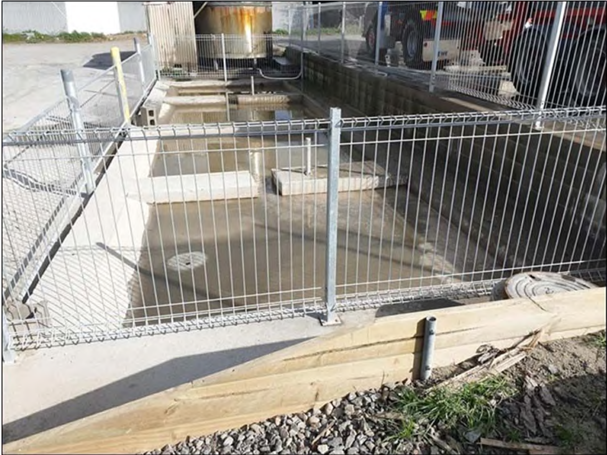
Photo 2 FBT truck wash discharge to trade waste
